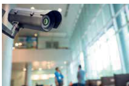
Security & Access Control
